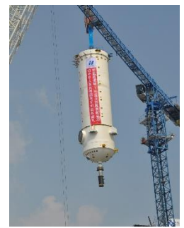
2016, RPVs on site and installed
