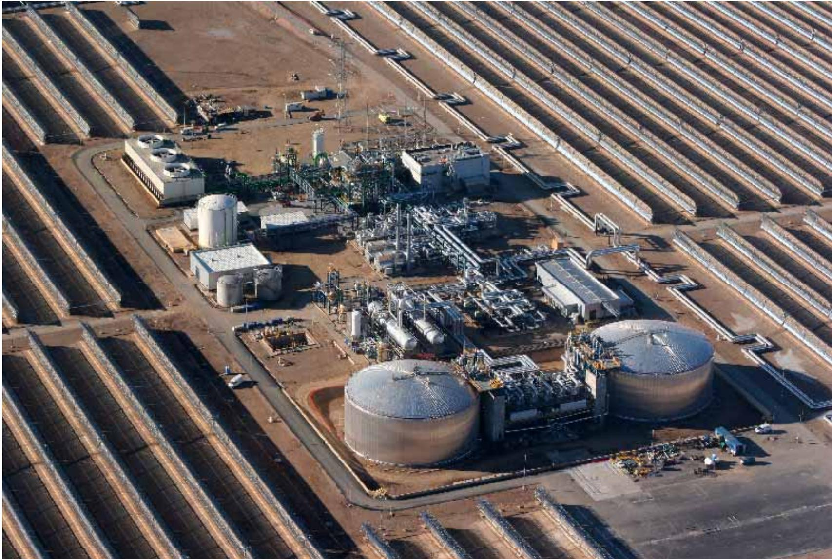
2 towers:  $\varnothing = 36 \text{ m}$ ;  $h = 14 \text{ m}$
